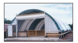
Ponywall Diamond Shelters come complete with rafter base couplers and lag bolts for wood, or optional wedge anchors for concrete.
